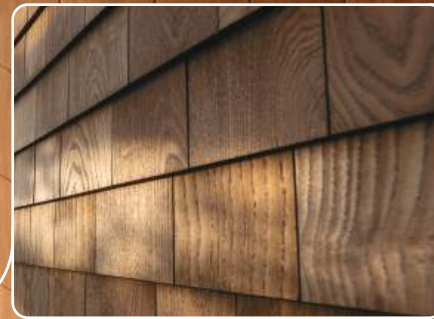
Shingles thermo-ash cladding
